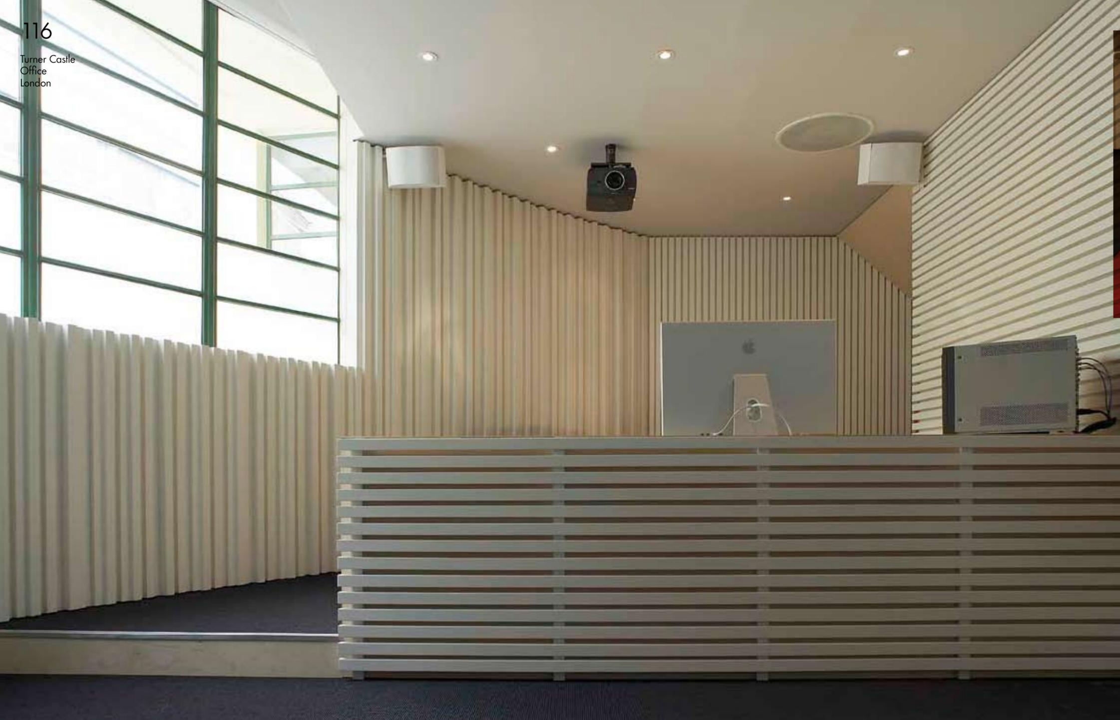
Pictured is an edit desk in the presentation edit suite, which is used for client viewings and functions as a small cinema. A split-level floor enables the editor to view the same screen as the audience (over their heads). Ridged wall surfaces help break up sound reflections to produce a better quality of sound.
